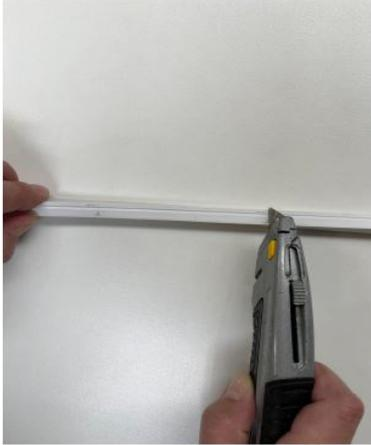
**Step 1:** Cut flex tape down to size on the nearest dotted cutting line.
